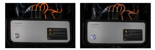
Make sure the electrical box is turned off by viewing the "start" button on the left hand side. The button will be a solid blue ring when on , and no color when off.
